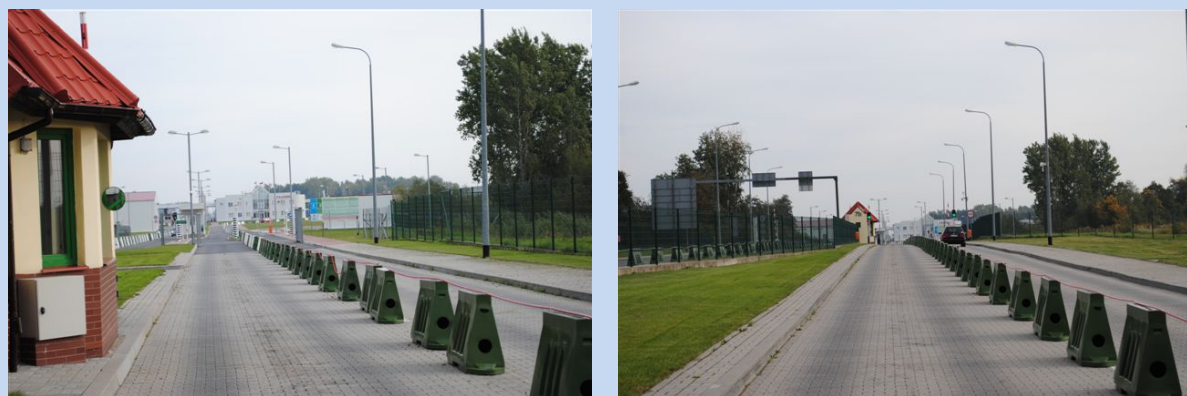
Photo 4 & Photo 5 Mobile separators for continuous green corridor
