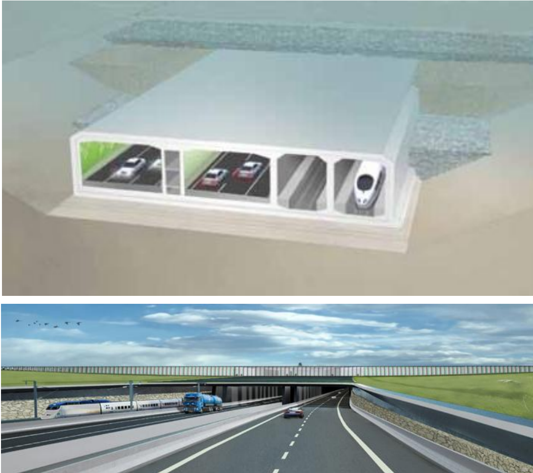
Figure 26. Cross section and entrance of the tunnel 49
