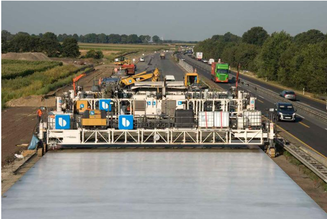
Figure 25. Construction of BAB 1 during traffic flow 29
