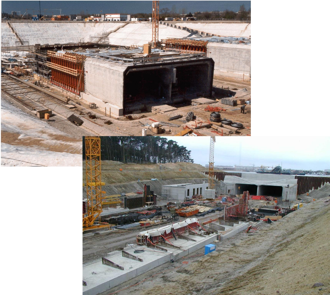
Figure 22. Building dock and eastern tunnel portal with dredger 16
