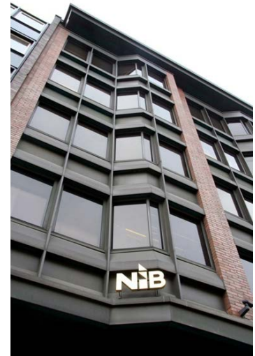
NIB Headquarters in Helsinki, Finland.
